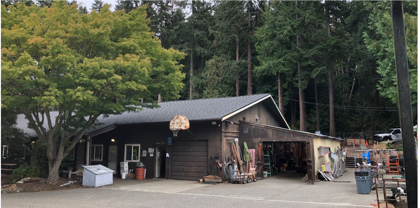
600 3 rd Avenue South, City Park
