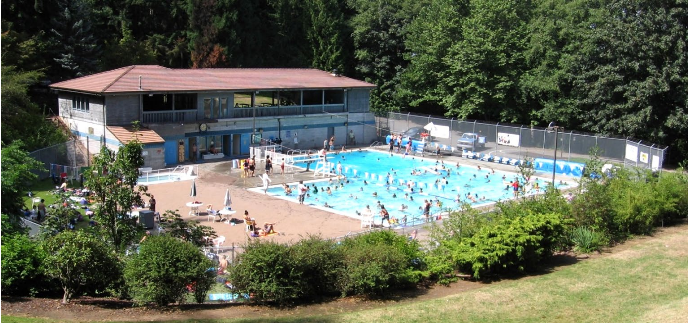
96th Ave W & Bowdoin Way, Yost Park
